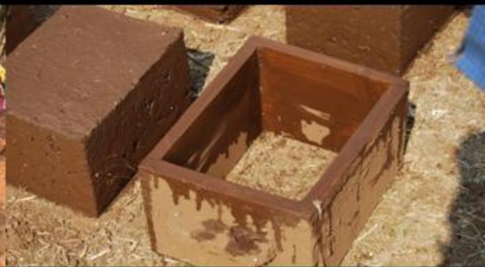
Mix a mix, wet the mould
