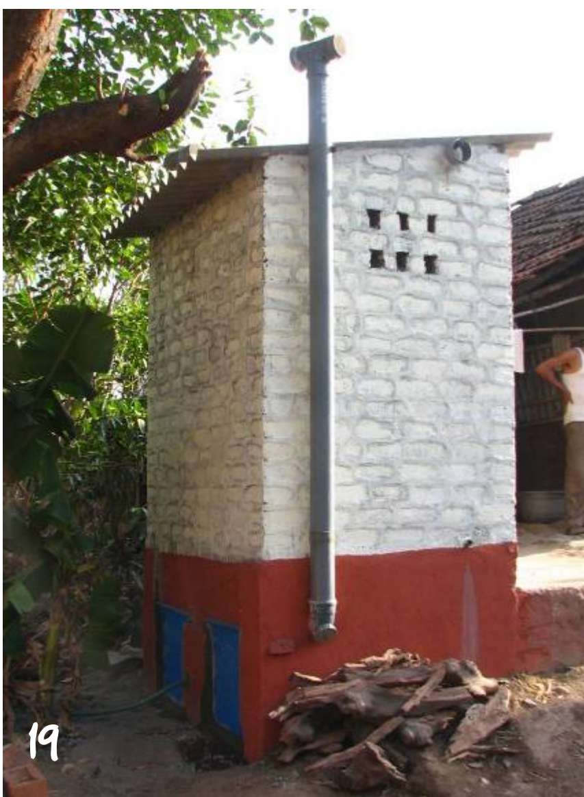
19: Vent pipes with mosquito nets at both ends. FRP sliding doors for chamber access. Pipe leads Urinet Wash water to bananas.
