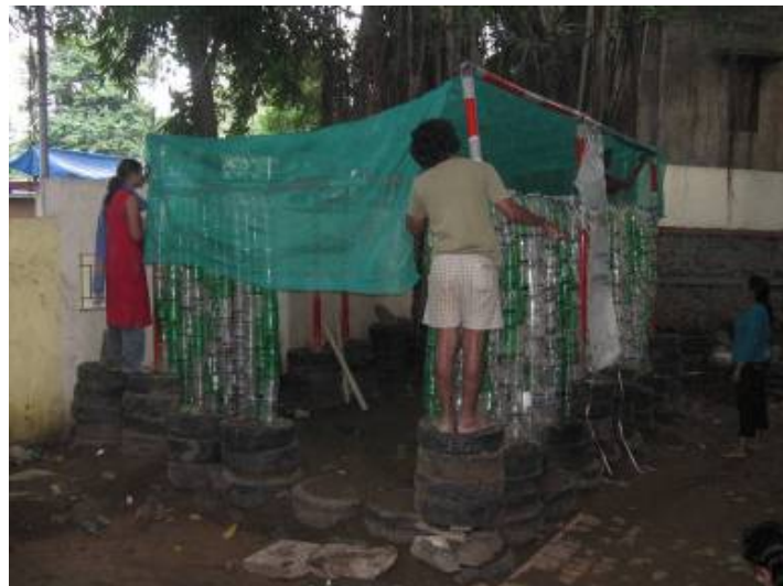
Post repairs, shade net to the rescue..
